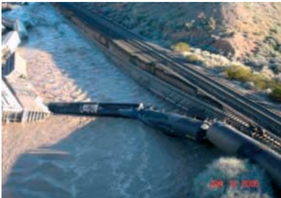
Flood disruption on the Union Pacific mainline, January 2005
